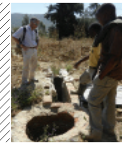
Fig. 158 Biogas system under construction
