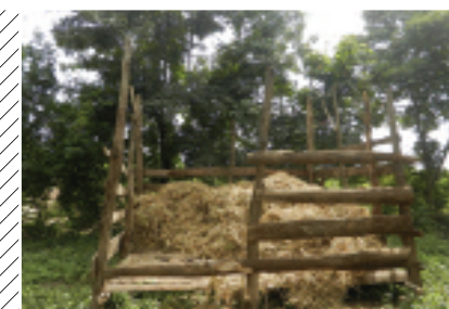
Fig. 137 Wooden storage structure for bean residues
