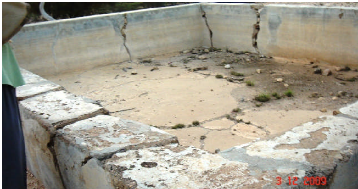
Broken water reservoirs Dabis River (GWX)
